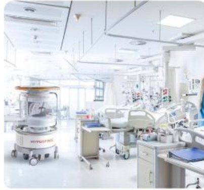
Intensive Care Units and Operating Rooms
